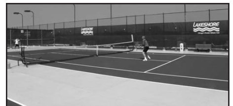
Photo 2 – The author designed this rooftop tennis court on the Lakeshore Athletic Club roof to serve a function besides just watertightness.
