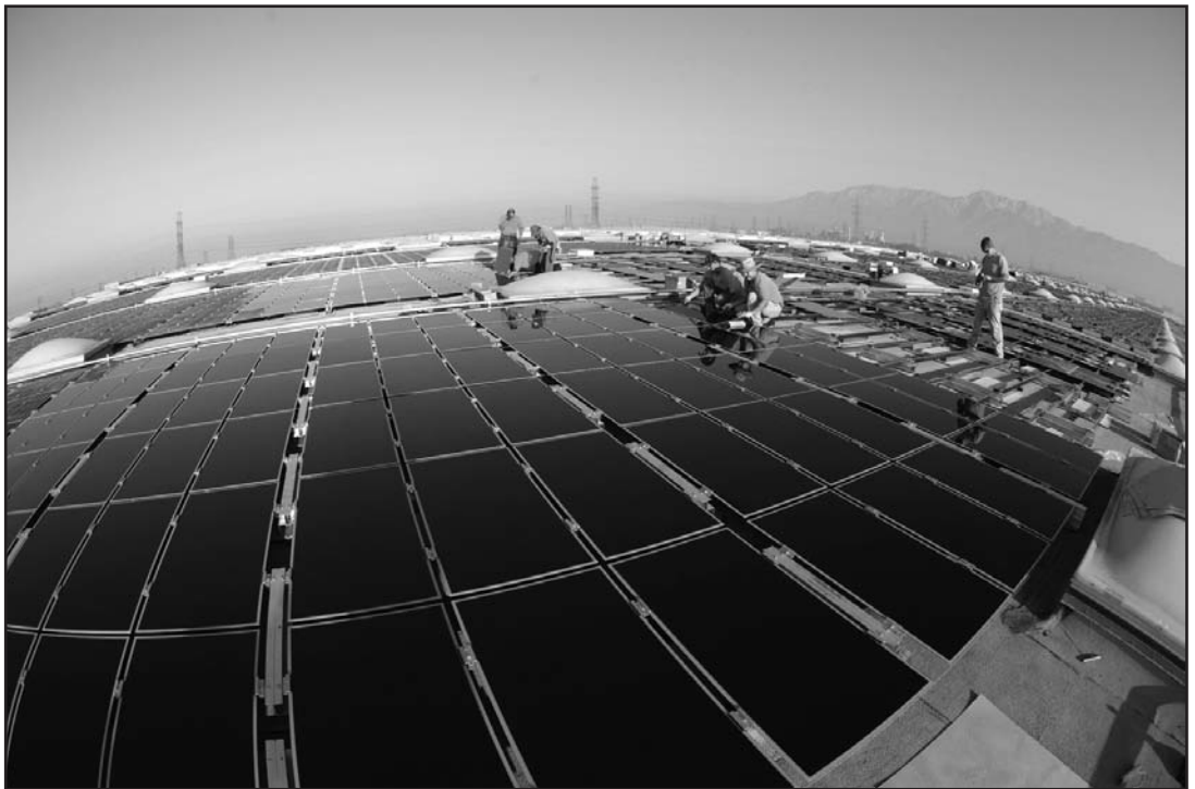
Photo 10 – This solar panel installation allows little room for maintenance of the roof surface below – a requirement of the roof warranty.
