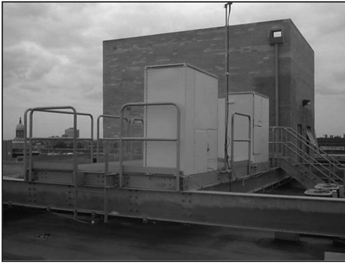
Photos 8A and 8B – Roofs have become prime candidates for the installation of cellular towers. As such, roofs need to be designed to accommodate for the installation and maintenance of the tower and the associated piping, cables, etc.
