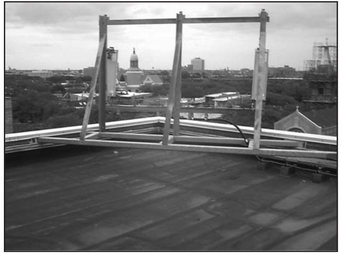
Photos 8A and 8B – Roofs have become prime candidates for the installation of cellular towers. As such, roofs need to be designed to accommodate for the installation and maintenance of the tower and the associated piping, cables, etc.
