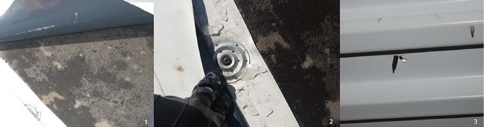
(1) Condensation below mechanically fastened cool-roof membranes in regions with cool nights is resulting in saturated insulation facers below the membrane. The results include mold growth, interior leaking and loss of wind-uplift performance caused by roof-deck corrosion. (2) Condensation below cool-roof membranes not only is saturating the insulation but resulting in ice build-up in the lap seams. (3) Moisture is dripping out of the errant screw hole. Repetitive wetting will result in roof-deck corrosion and, when located at screw fasteners, loss of wind-uplift resistance.
